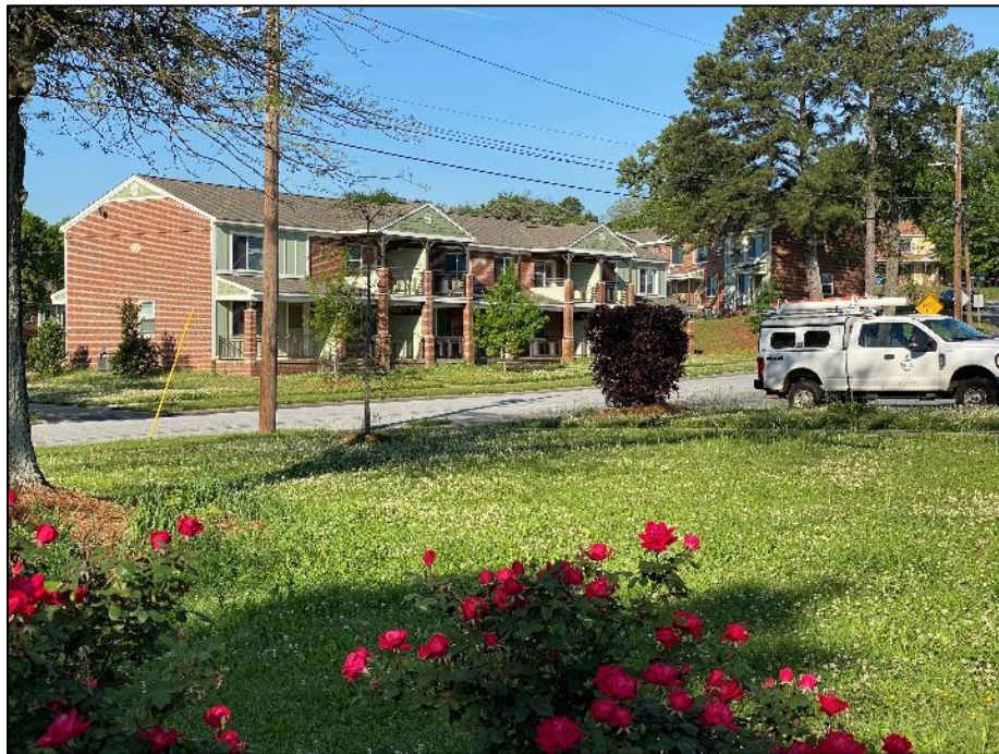
Figure 38: View from Community Center towards FS
